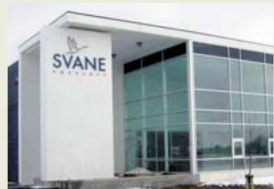
Svane Logistik Center A/S outside Vejle in Denmark.
